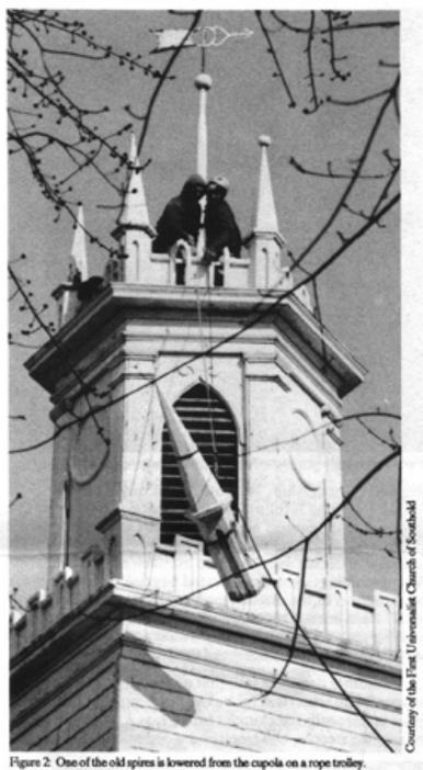
Figure 2. One of the old spires is lowered from the cupola on a rope trolley.
