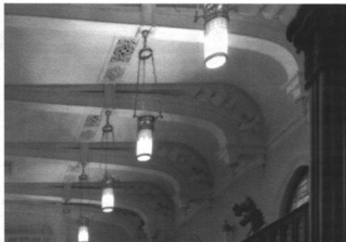
The sanctuary of St. Stephen's Episcopal Church, 10th Street below Market Street, is equipped with ornate grilles that run in parallel rows like this one along the ceiling. This system, which has been used since the 1920s to ventilate the building, may be used by the congregation in the near future to implement central air-conditioning. Detail of photo: William Douds Photography.
