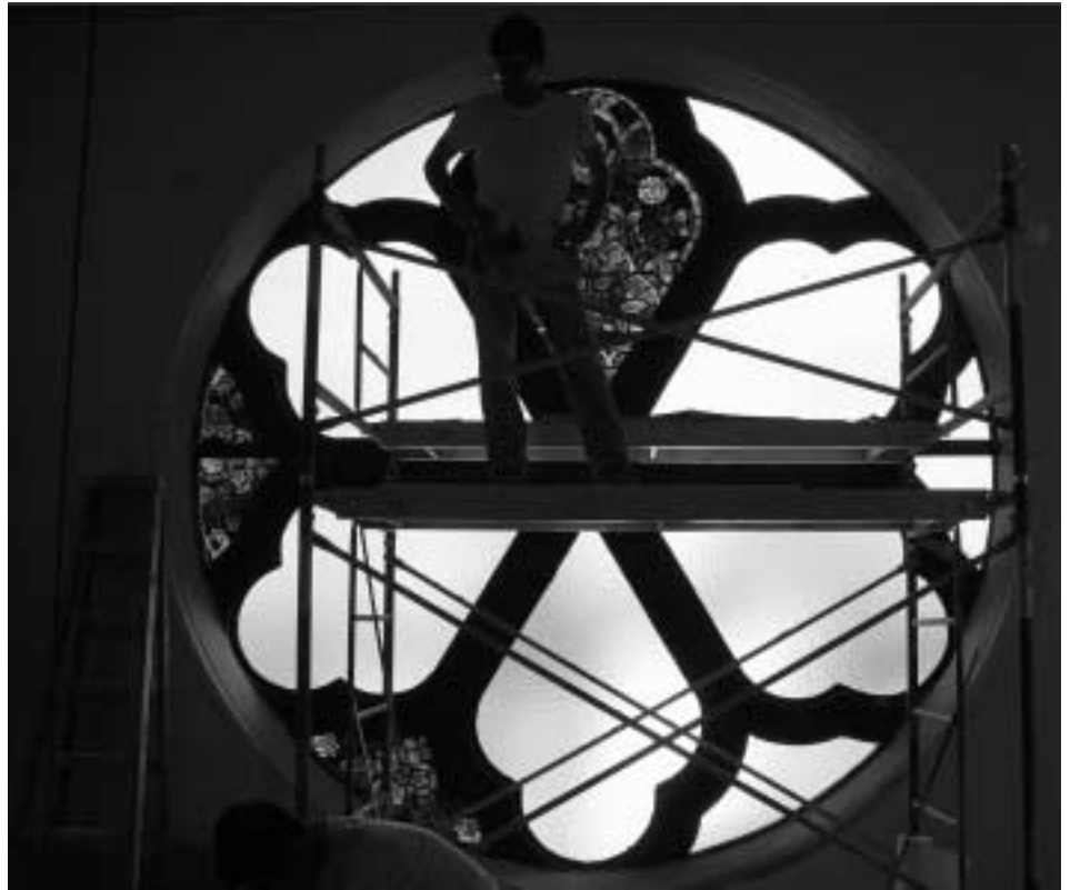
Rambusch employees installing a stained glass window.
