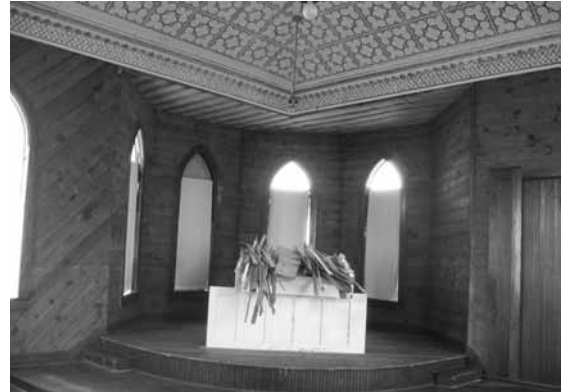
The plaster removal process in the summer of 2007 uncovered a beautiful piece of history. The Swedish craftsmen used high-quality wood, placed at angles, to provide a solid structure for the church.
