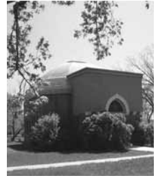
Historic Isaac Solomon Synagogue was built in 1926 on the grounds of the Jewish Consumptives' Relief Society in Lakewood, Colorado.
