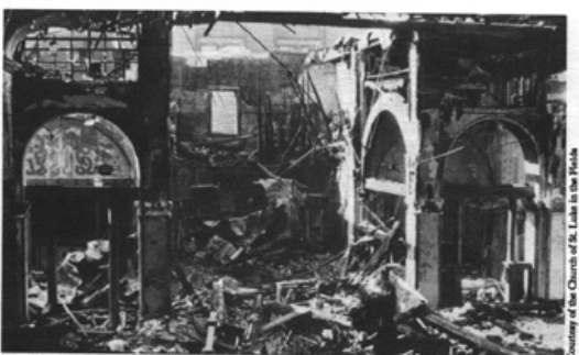
Figure 3: The Interior the Day After the Fire
