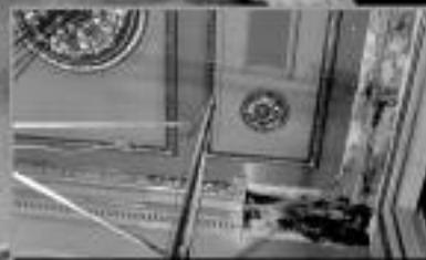
PLASTER & PAINT RESTORATION
